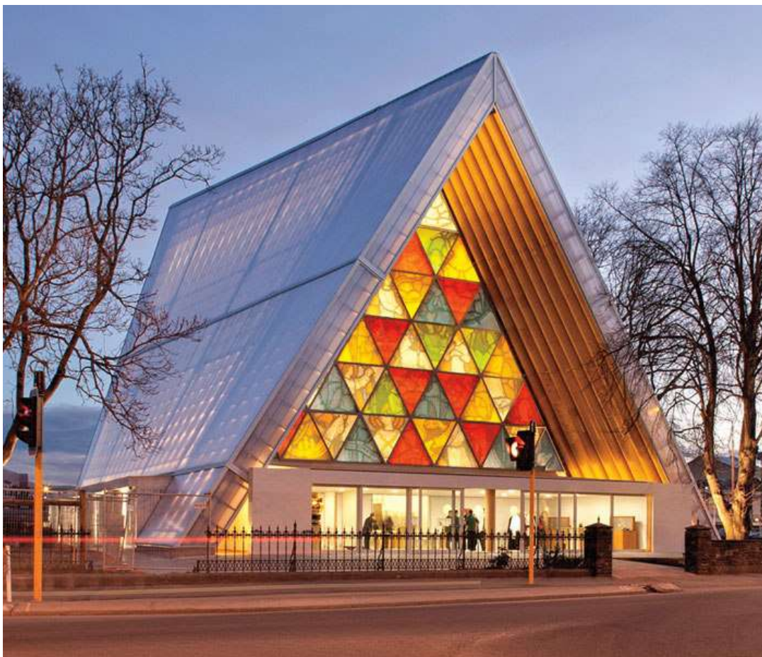
The transitional cardboard cathedral in Christchurch, New Zealand. In the picture we can observe the non-planarity of the lateral face due to the difference of width between the front and back triangular faces. http://www.addingtonbrass.com/wp-content/uploads/2015/06/Christchurch-Cathedral.jpg
