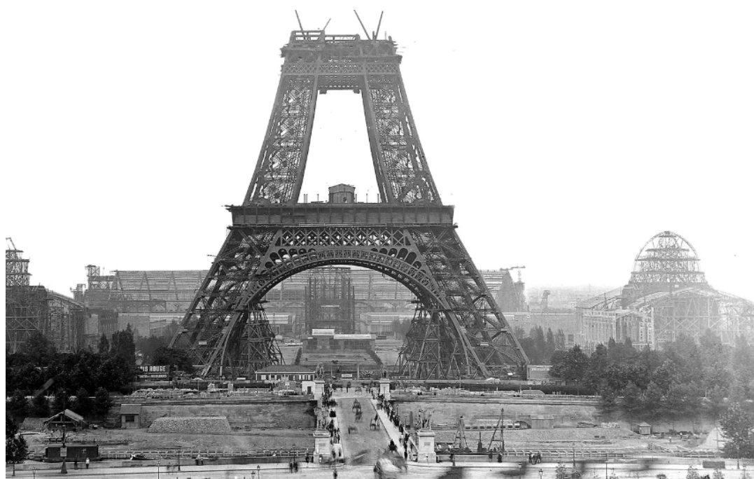
The Eiffel Tower under construction in July 1888. Roger Violette/Getty Images
