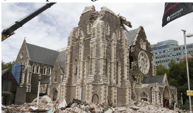
Shortly after the earthquake, 22 February 2011 (www.newshub.co.nz)
